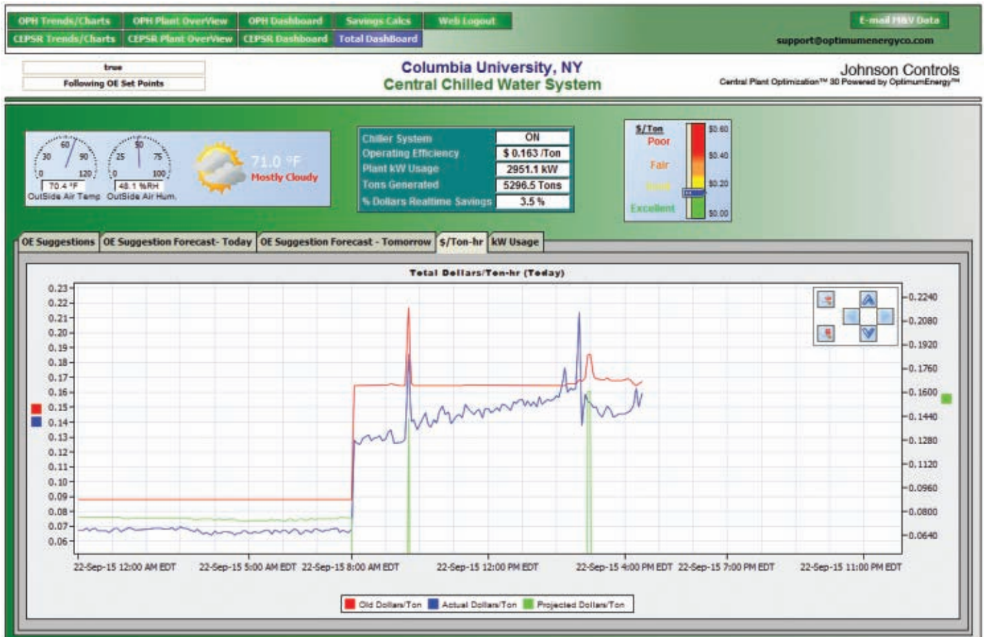
Figure 3. Screenshot of Total Dashboard View, OptimumLOOP Platform, Central Chilled-Water System, Columbia University.
